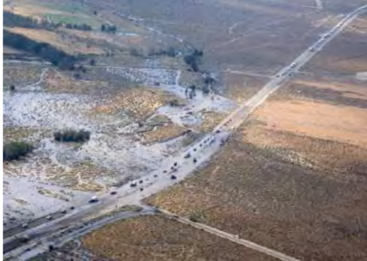
Mud flowing across Highway 395 requiring CHP escorts to guide traffic through.
